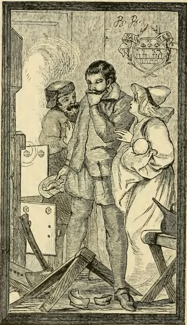
HEATING THE FURNACE.
